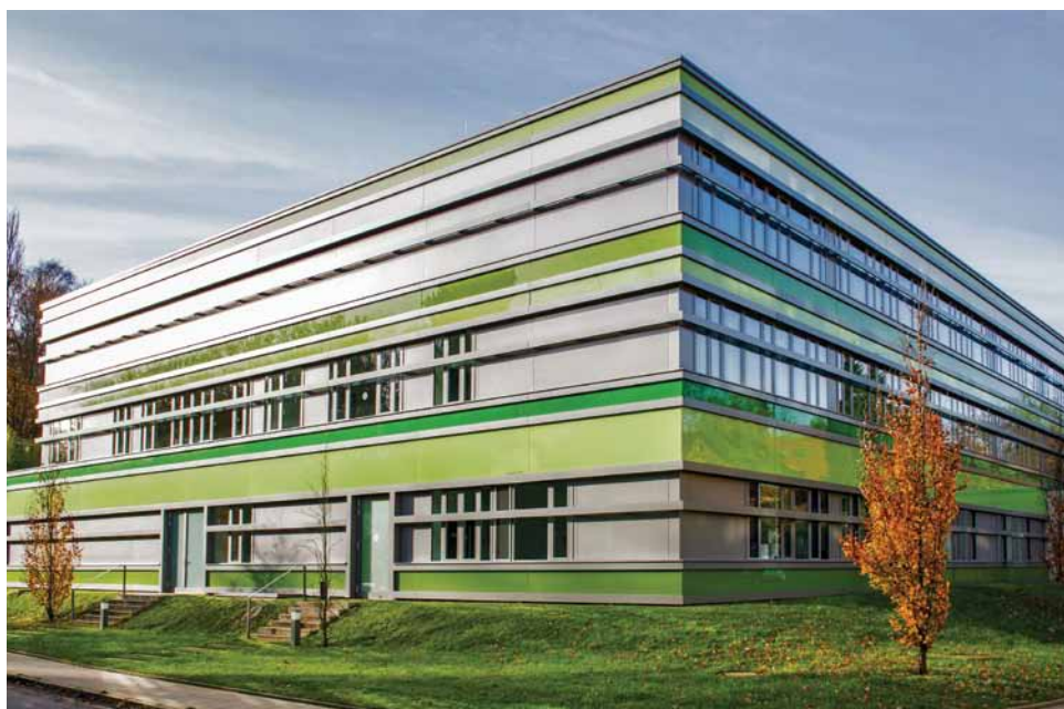
Fig. 4: Building of the WPE facility (reference: WPE)
